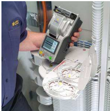
Figure 2: Coupler Splice-in
